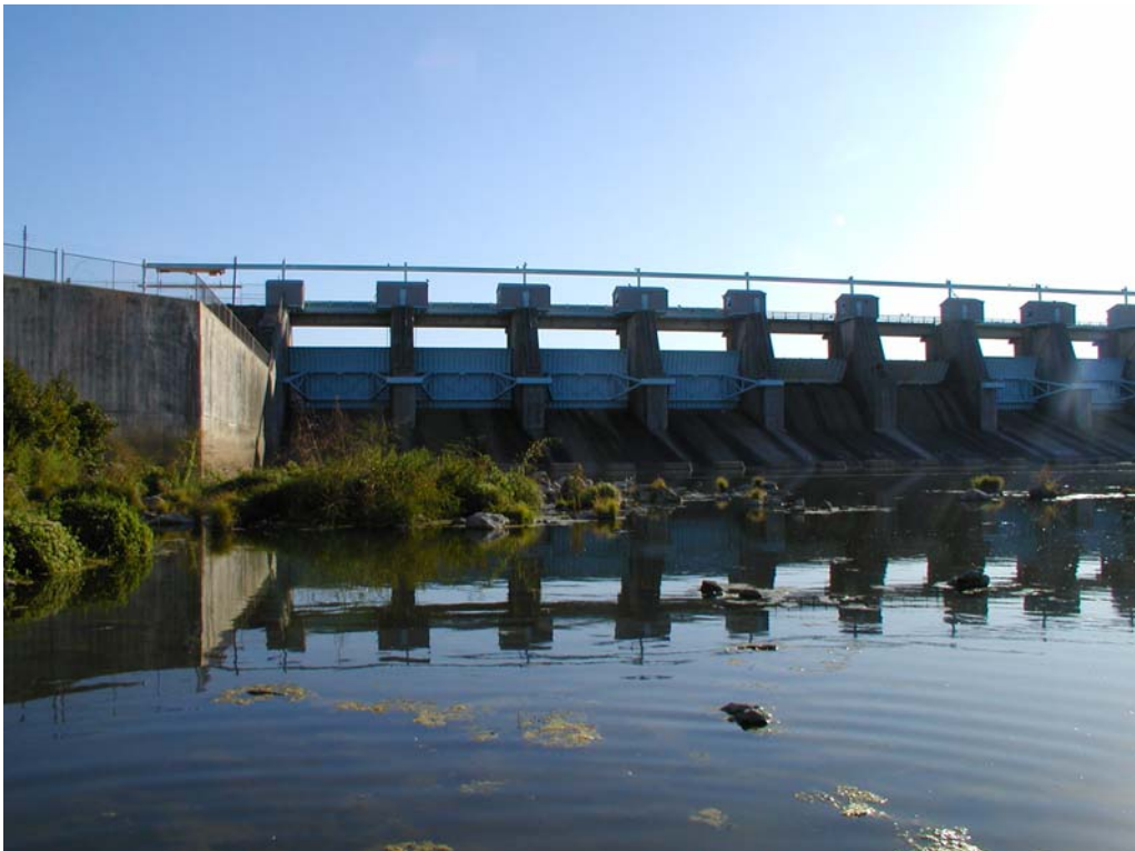
Figure 3-32. Cedar Creek Reservoir Dam
