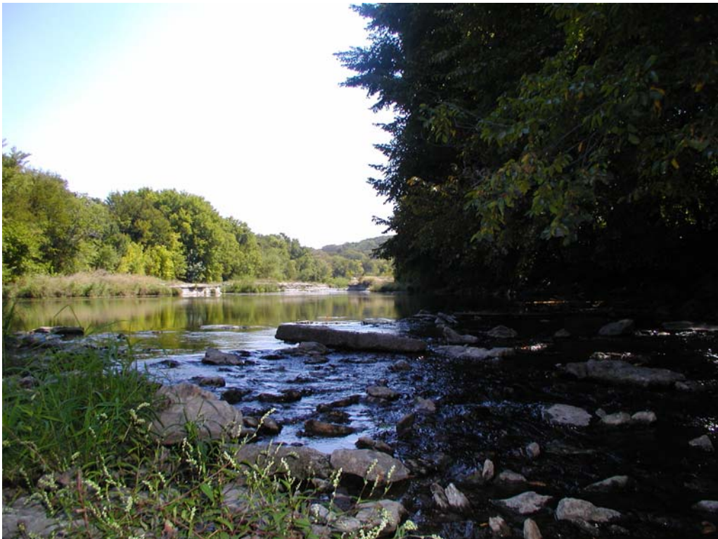
Figure 3-24. Benbrook Reservoir Stilling Basin Downstream
