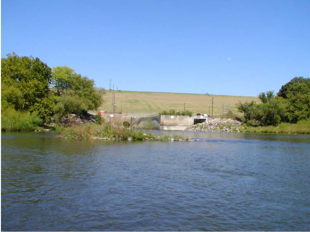
Figure 3-29. Lake Lewisville Stilling Basin
