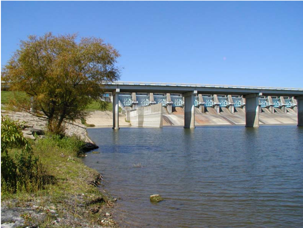
Figure 3-33. Richland-Chambers Reservoir Stilling Basin
