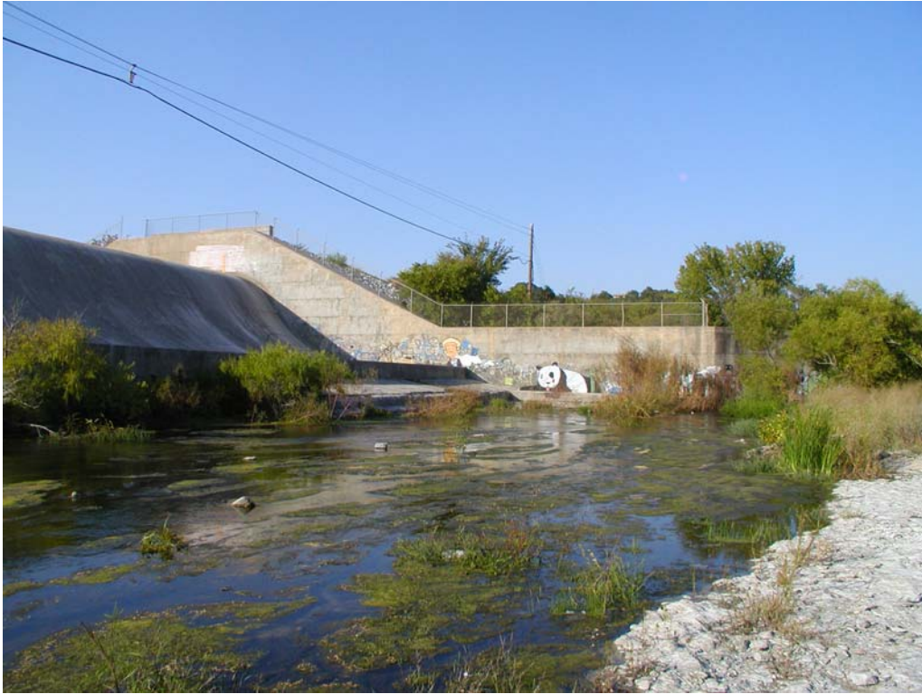
Figure 3-25. Lake Worth Dam and Stilling Basin
