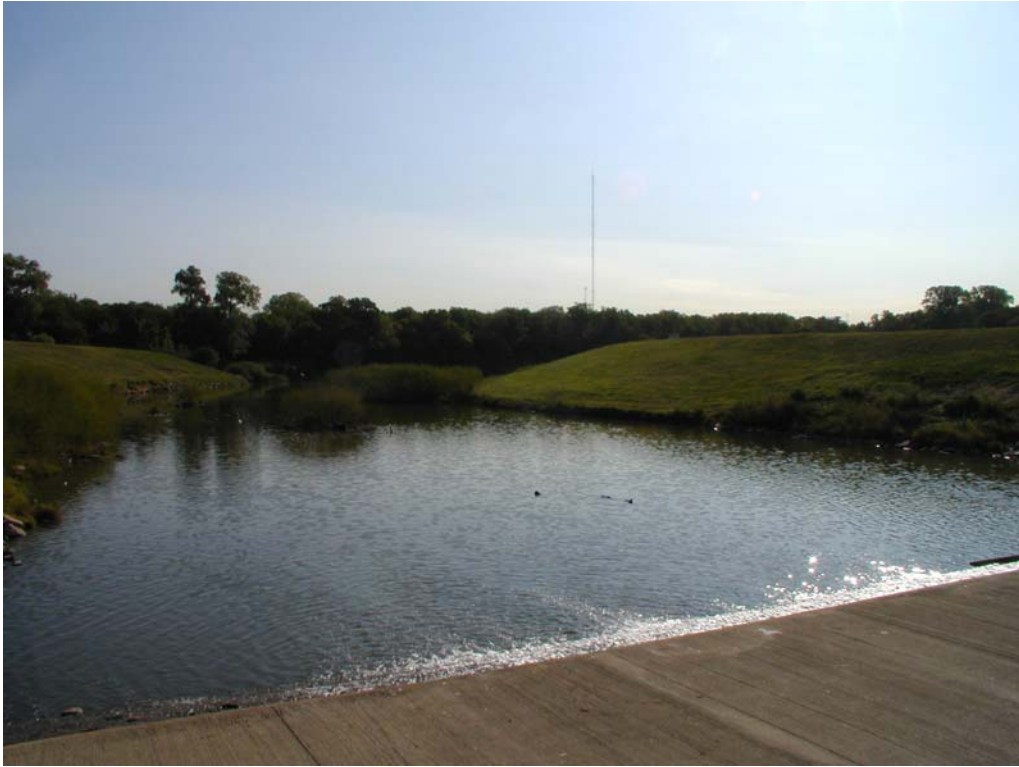
Figure 3-27. West Fork Trinity River at Beach Street
